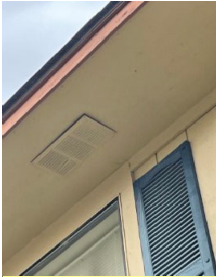
Soffit and Fascia
